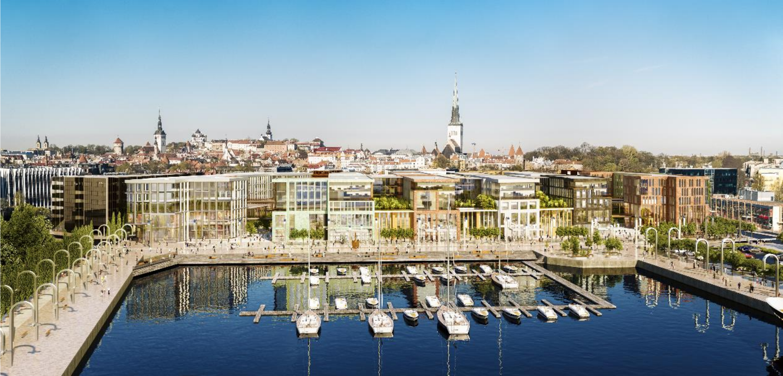
New Campus – Porto Franco in Tallinn in fall 2020
