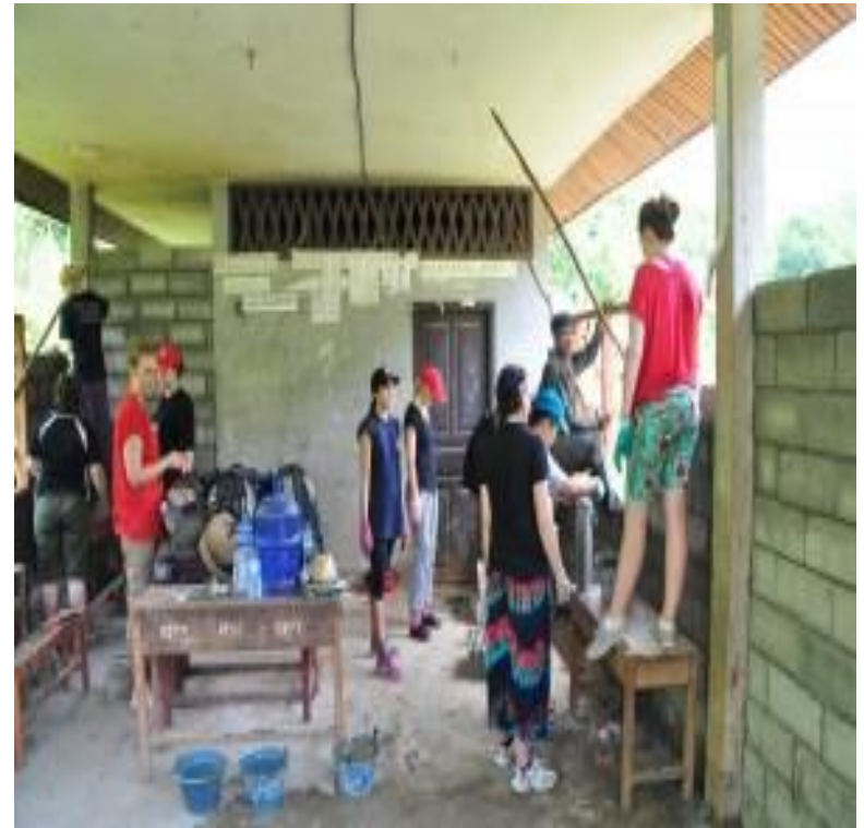
Renovating a high school classroom
